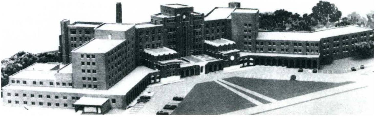
Aerial view of Saint Cloud Hospital, ca. 1965. Photo from the Stearns History Museum and Research Center archives.
